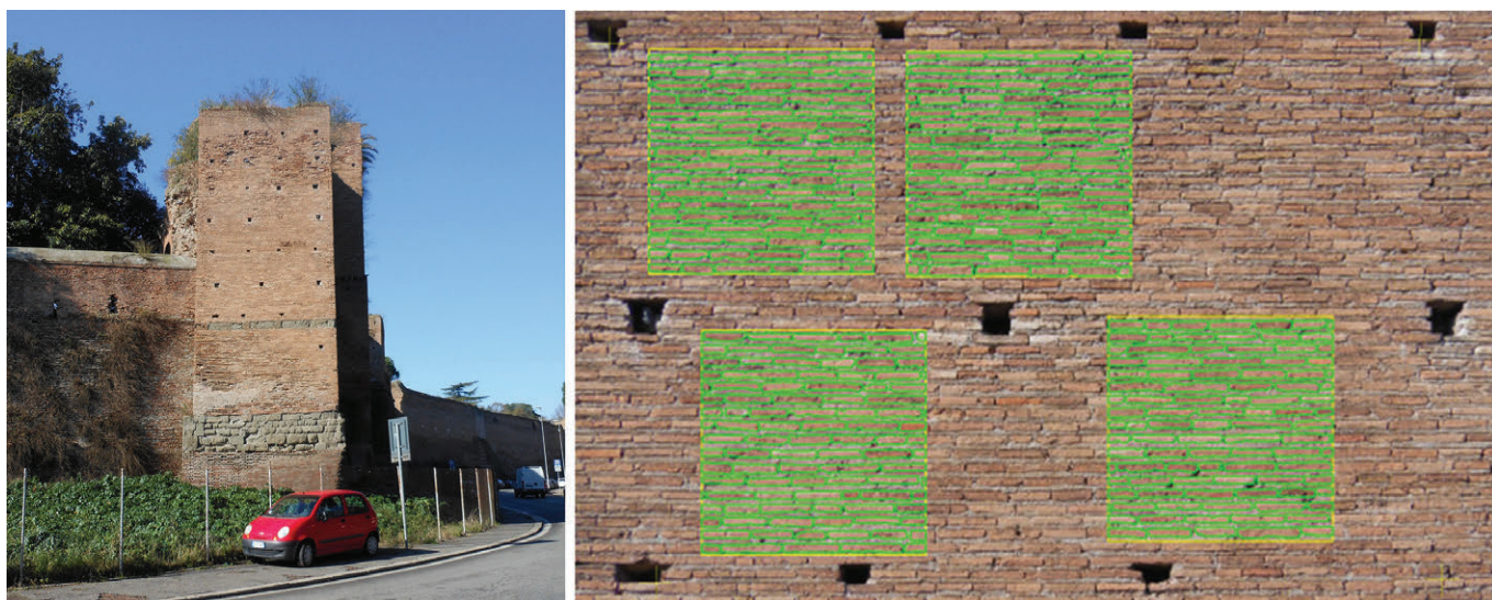
Fig. 4. Aurelian Walls, sampling of tower K07. Right: general view; left: central side, samples 01-04.
